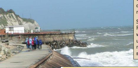
Concrete walls or rock structures built along a stretch of coastline and designed to stop erosion and floods. Sea walls reflect waves, and give complete protection against erosion.
